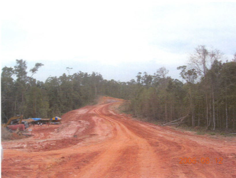
Over-designed road to northern resettlement villages
