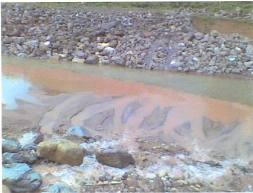
Powerhouse discharge flowing directly into Nam Kathang
