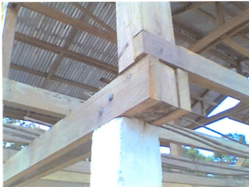
Solid resettlement house frames, new Ban Sop On
