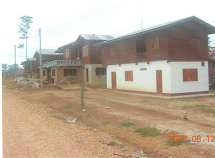
Owners are modifying some resettlement houses---one with basement area enclosed, a second being converted into a tavern as well as a dwelling. Saddle Dam, Nakai
