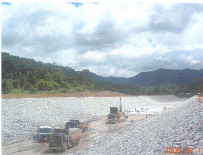
Lining the substantial downstream channel
