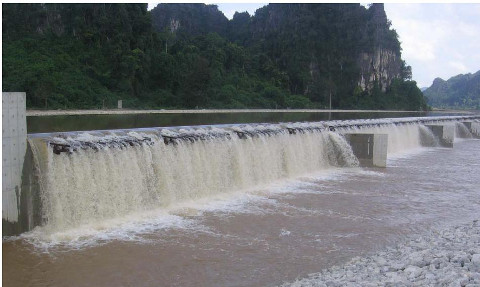
**Fig. 4.** Picture of the aerating weir downstream of the regulating dam in the Downstream Channel.
