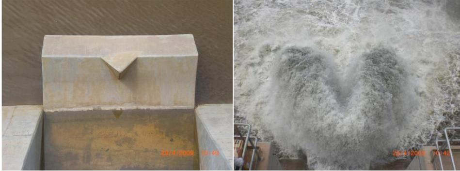
**Fig. 3.** Picture of the concrete tooth shaped structure downstream of the Regulating Dam in the Nam Kathang River.
