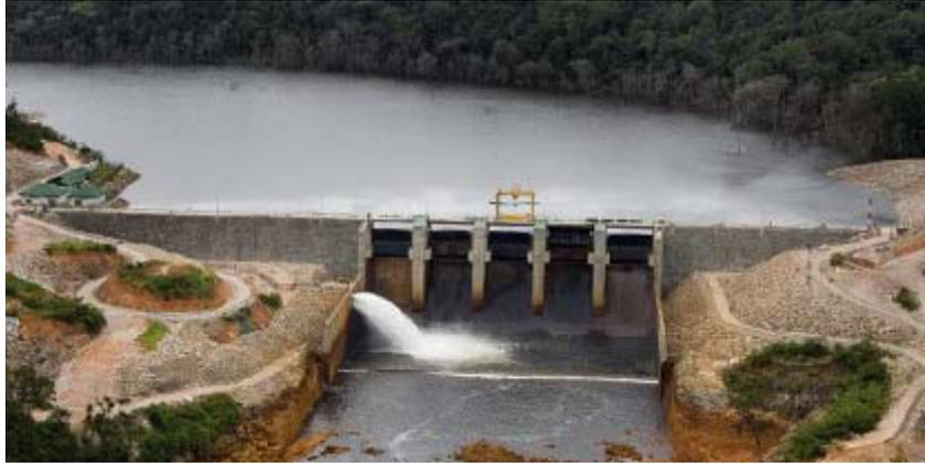
**Fig. 1.** Picture of the riparian release structure of the Nakai dam site on the Nam Theun River (hollow jet valve).
