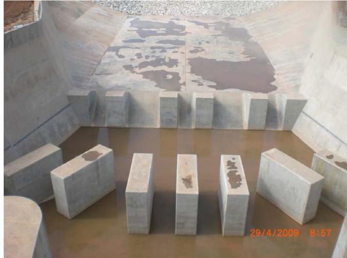
**Fig. 2.** Picture of the staggered baffle blocks installed downstream of the Regulating Dam in a convergent section in the Downstream Channel.
