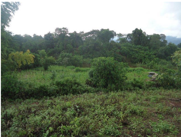
South/south east of the spillway construction area – Mr. Khamkong, Mr. Dii and Mr. Champa
